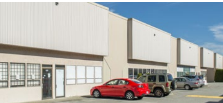
1776 BROADWAY STREET, PORT COQUITLAM, BC
