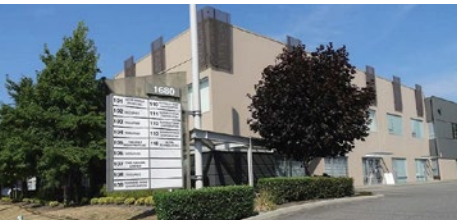
1680 BROADWAY STREET PORT COQUITLAM, BC
