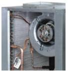
Dual compressor vibration isolation for quiet operation
